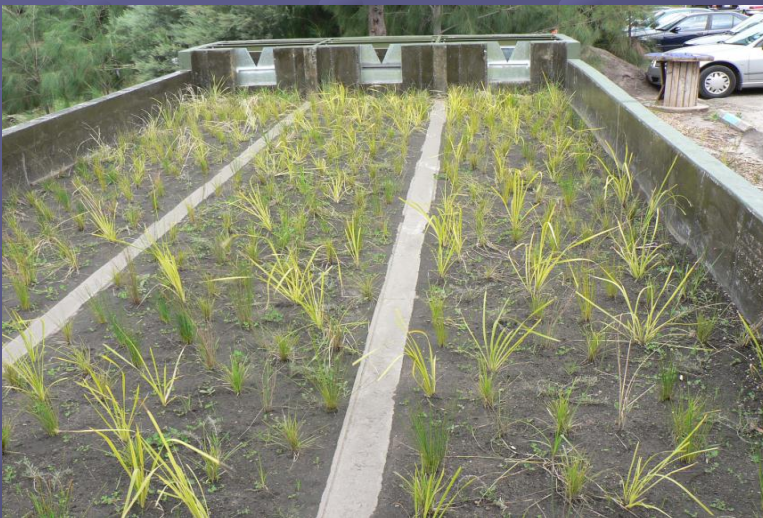
Horizontal Subsurface Flow-Sewage Treatment Wetlands
