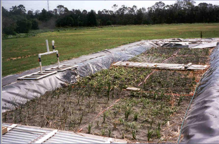
Horizontal Subsurface Flow-Sewage Treatment Wetlands
