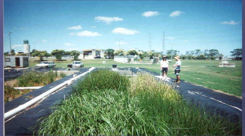
Horizontal Subsurface Flow-Sewage Treatment Wetlands
